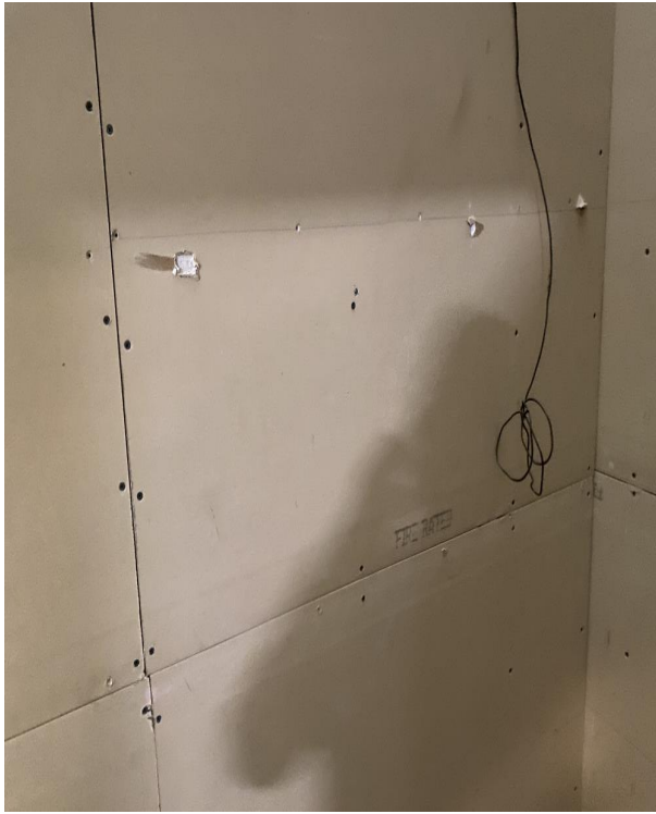
Photo 17 Comments: Drywall sample in thrift shop electronics room
