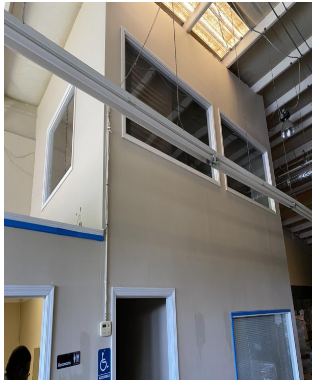
Photo 8 Comments: Fluorescent light fixtures in storage area
