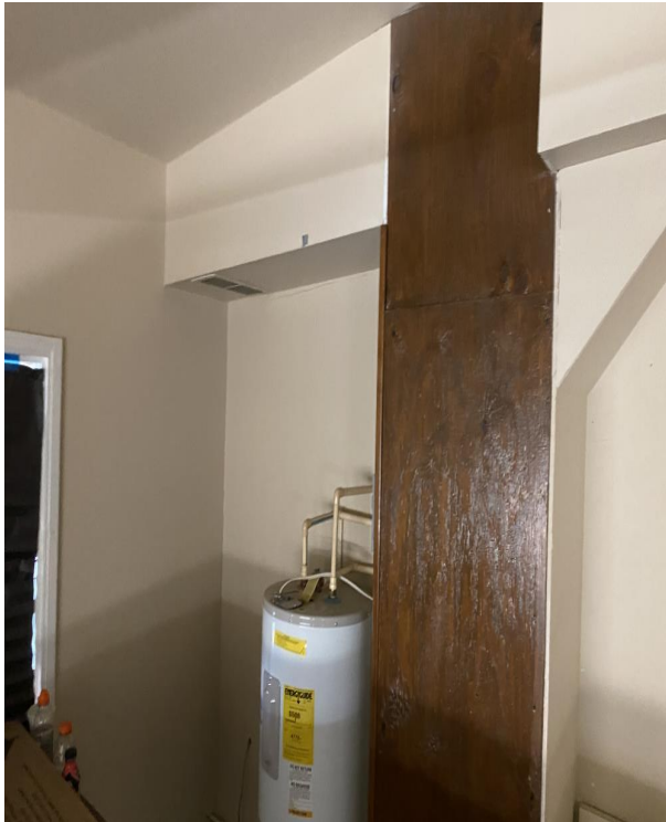
Photo 27 Comments: Storage room second floor
