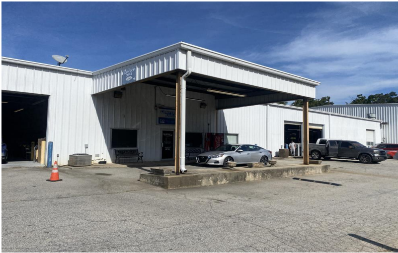
Photo 1 Comments: Main entrance
