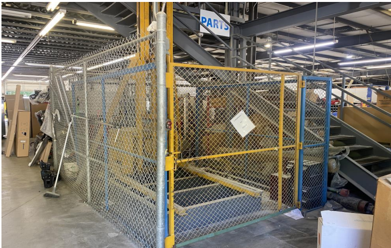
Photo 19 Comments: Lift to second floor
