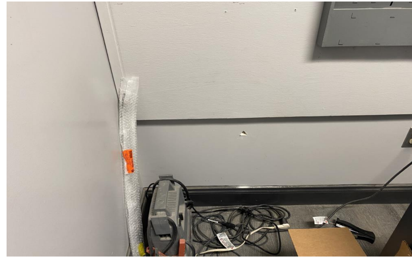
Photo 22 Comments: Office drywall sample
