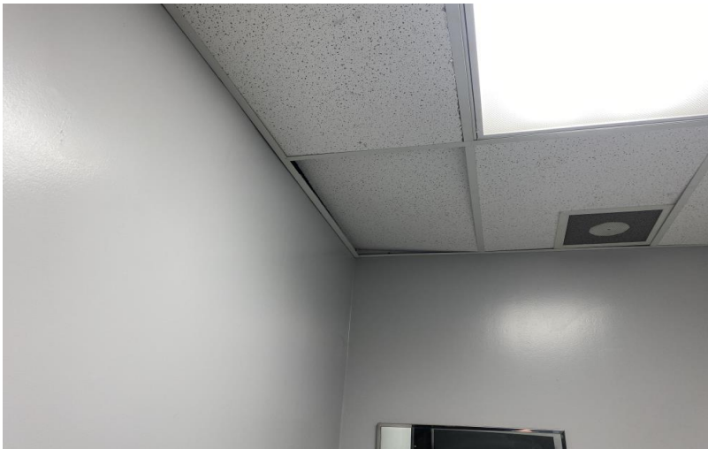
Photo 7 Comments: Office ceiling tiles
