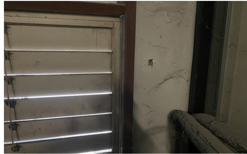
Photo 6 Comments: Wall insulation sample
