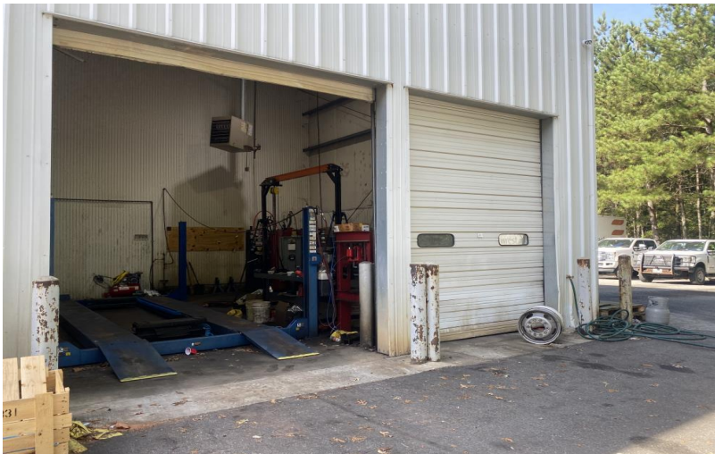
Photo 11 Comments: Diesel area east exterior
