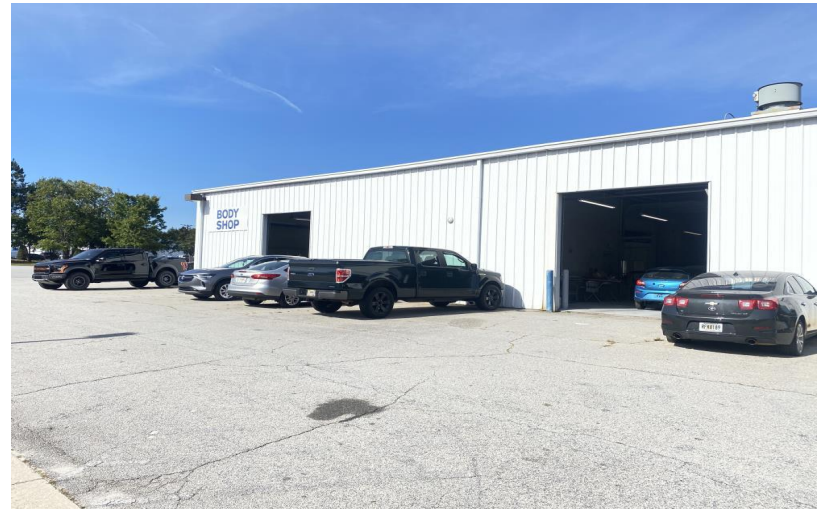
Photo 2 Comments: Paint area south exterior
