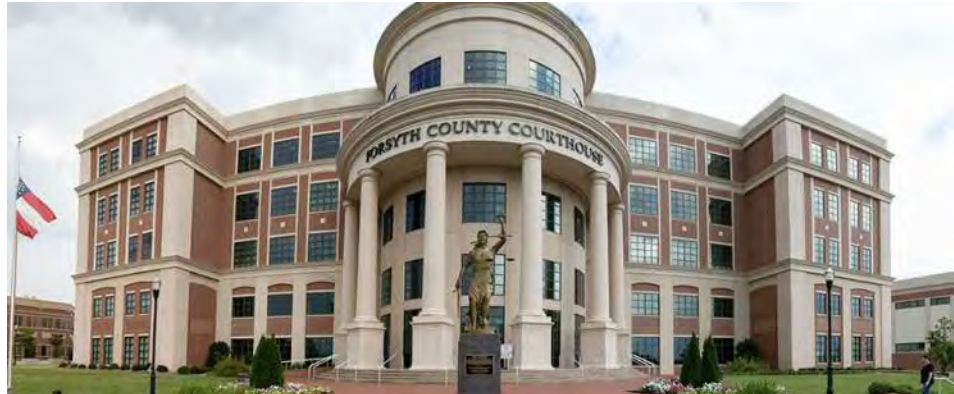
FORSYTH COUNTY COURTHOUSE
