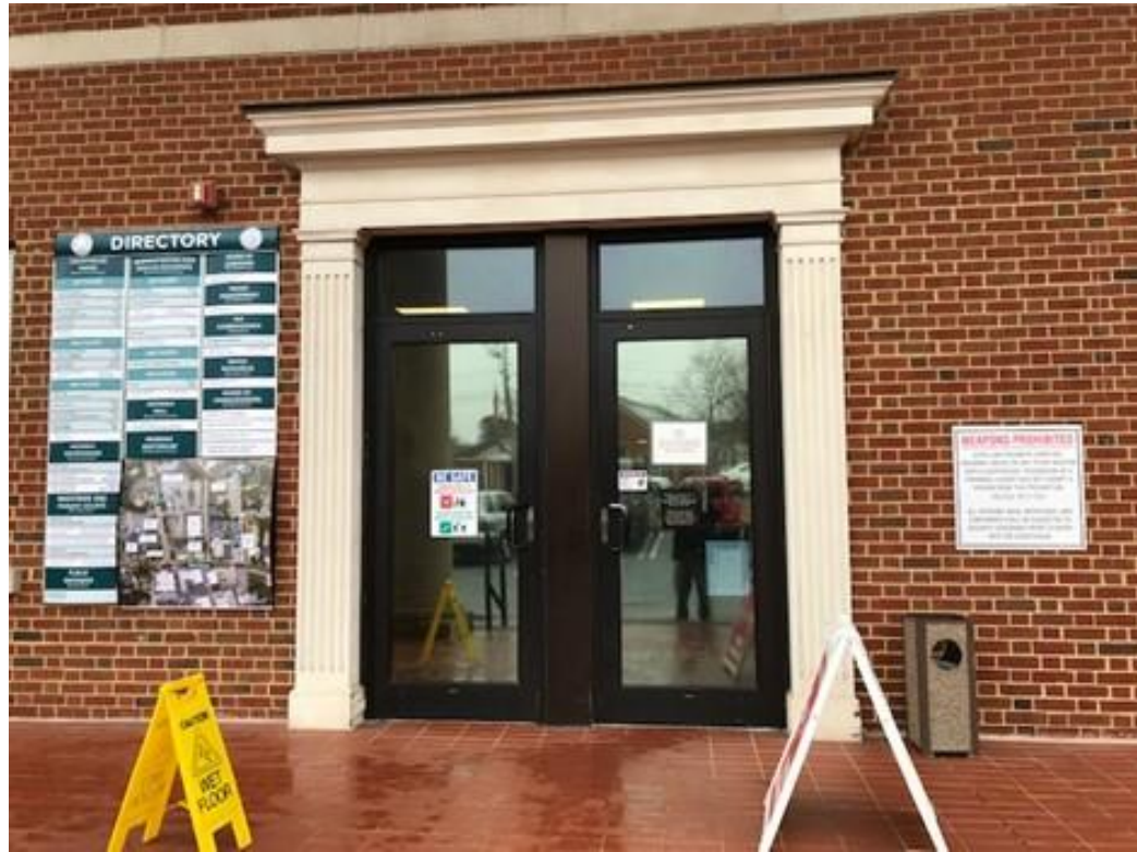
Item #8 -Storefront Entrance to be replaced *922 Court St Building view of windows
