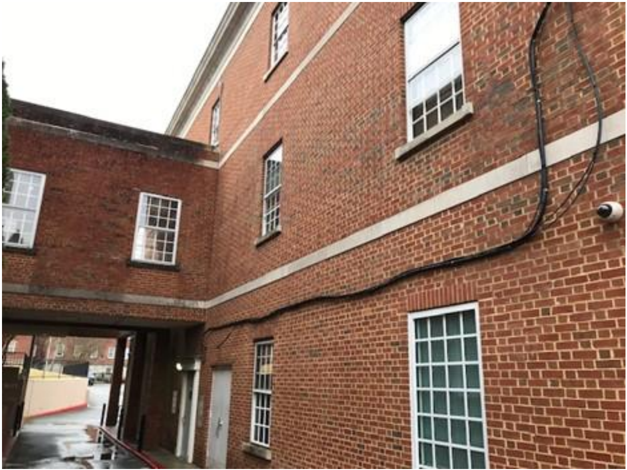
*Sallyport (South) view of building windows
