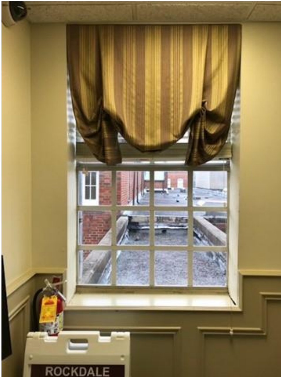
Item #6 - 3 rd Floor Window to be replaced with Operable Casement window for Roof Access
