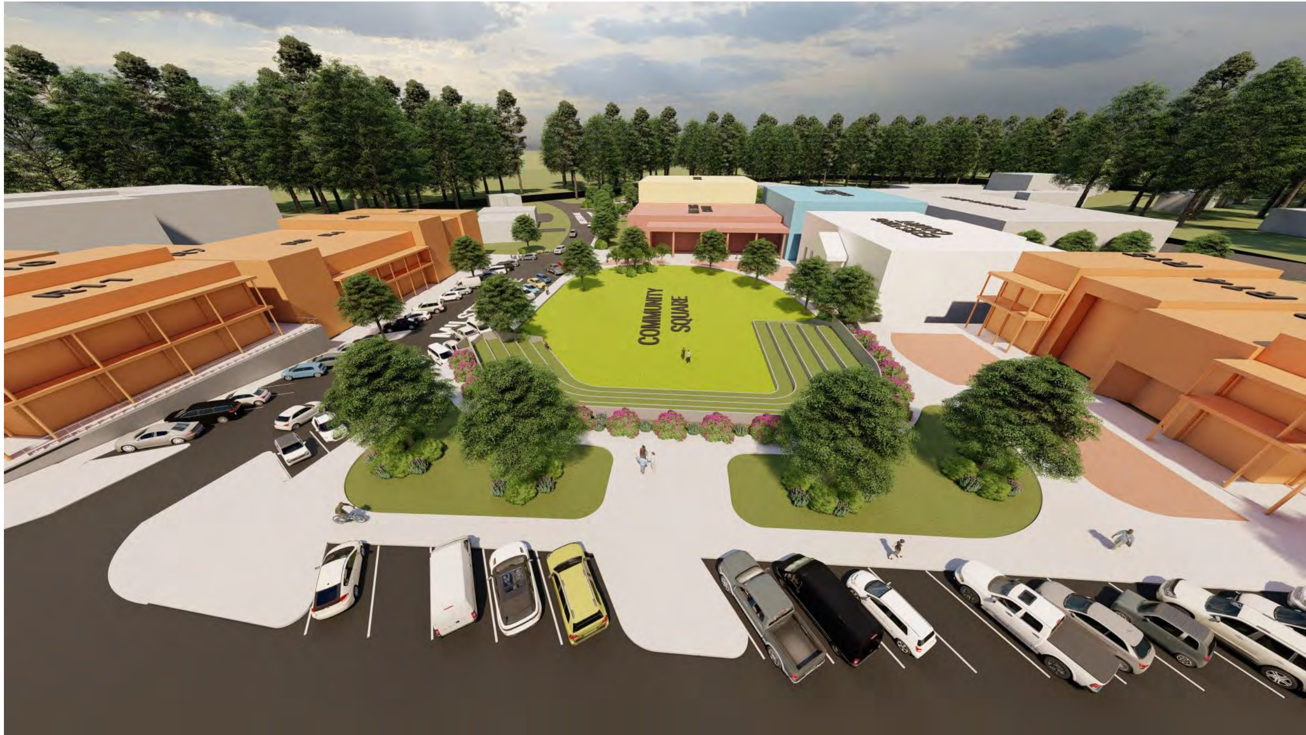
ROCKDALE COUNTY "COURTS & COMMUNITY ADMINISTRATION CENTER"
